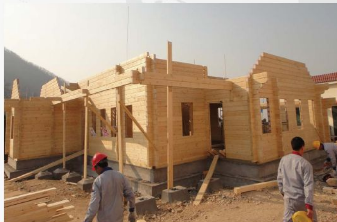
INSTALLATION WALL WOOD HOUSE
