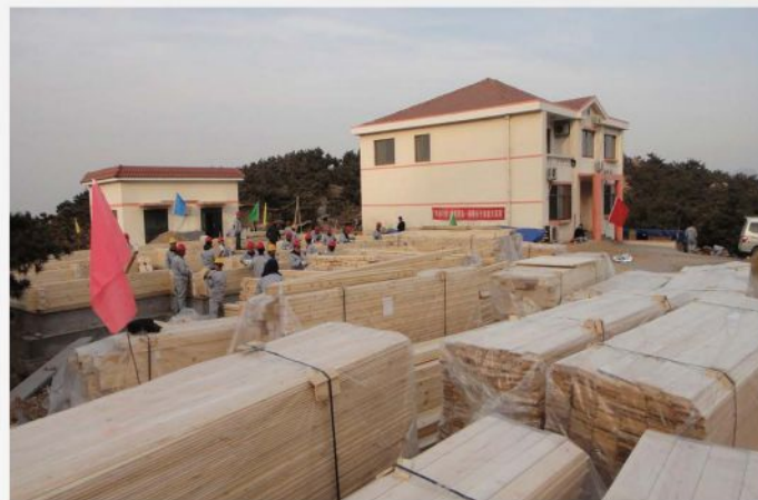
MATERIAL ON SITE WOOD HOUSE
